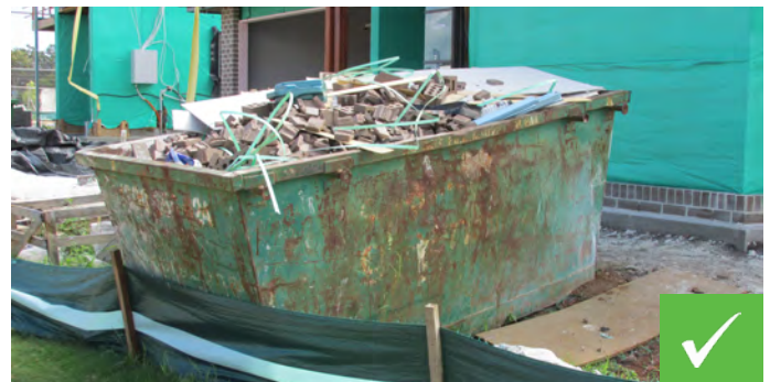
Keep all rubbish in covered skip bins or mesh cages (Source: Healthy Land & Water).
