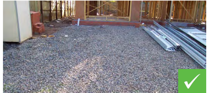
Entry/exit rock pad (Source: Brisbane City Council).
