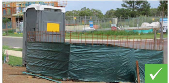
Fabric wrapped mesh cage (Source: Healthy Land & Water).
