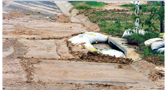
Stormwater inlet coarse sediment protection (Source: Brisbane City Council).
