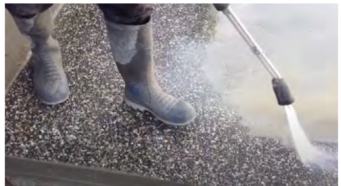
Exposed aggregate driveway (Source: Catchments & Creeks).
