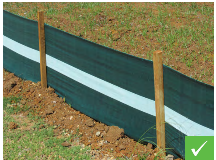
Sediment fence correctly installed (Source: Healthy Land & Water).
