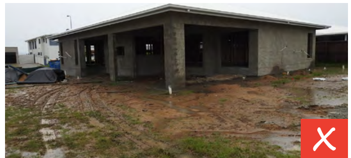
Erosion of site without rock pad (Source: Healthy Land & Water).
