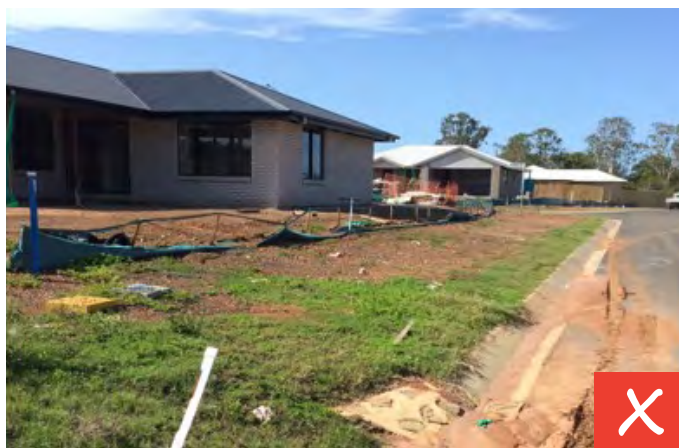
Site without adequate kerb to lot cover (Source: Healthy Land & Water).
