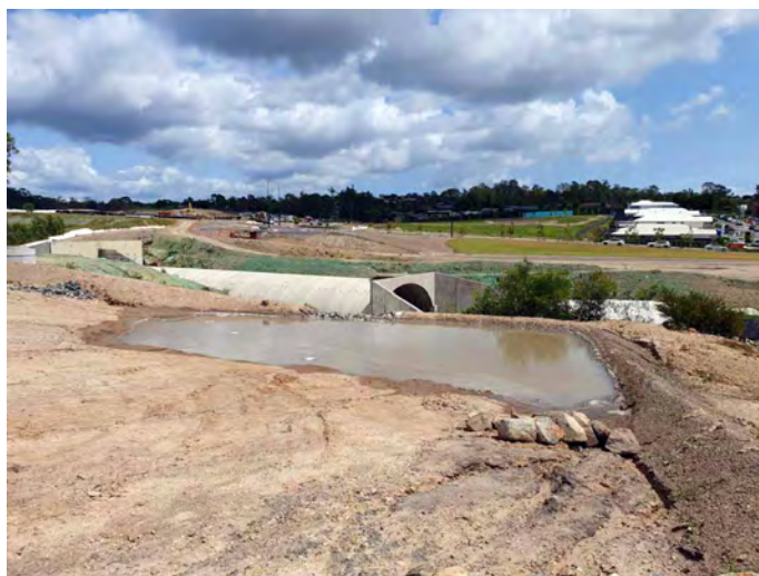
Excavated sediment trap (Source: Topo Group).
