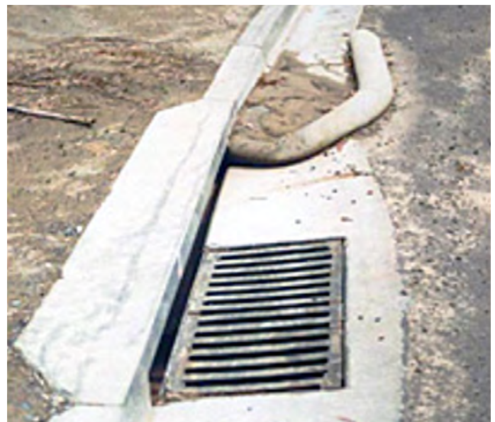
Stormwater inlet coarse sediment protection (Source: Brisbane City Council).
