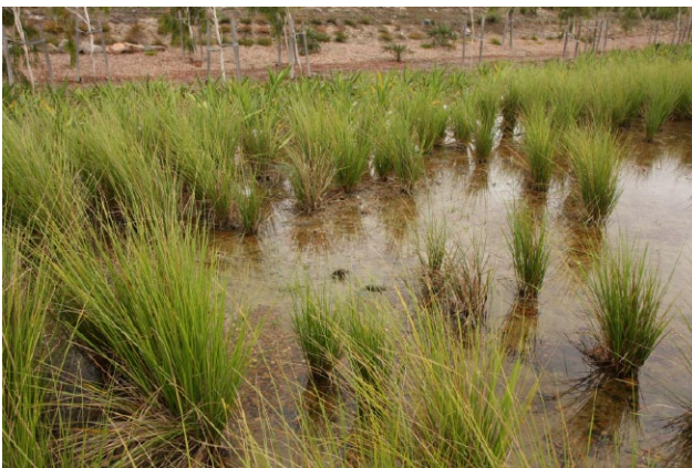
Figure 10 Bioretention system with water ponded on the surface
