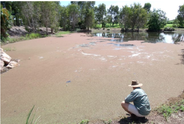
Figure 33 A sediment basin that is infested with floating weeds and lacks vegetation cover on the batters
