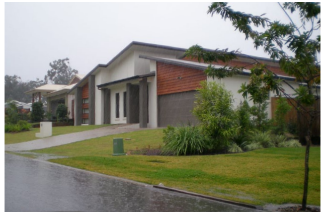
Figure 4 Localised flooding due to the swale being partially filled in
