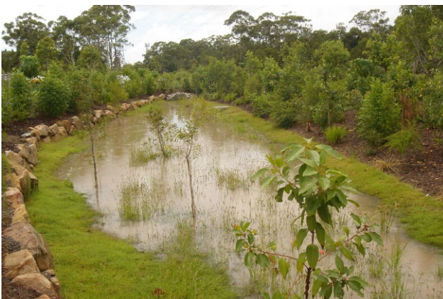
Figure 12 Bioretention system subject to backwatering: the surface level has been set below the level of the downstream receiving waterway
