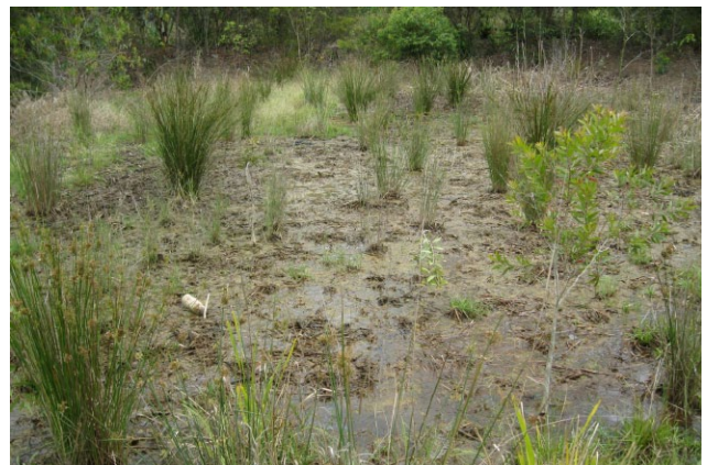
Figure 11 Bioretention system with water ponded on the surface due to inappropriate filter media
