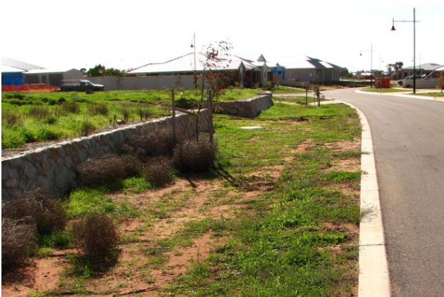
Figure 5 Swale with excessive sediment
