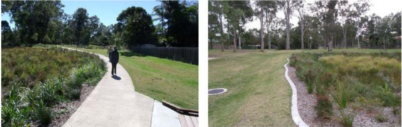
Figure 61. Maintenance edges to bioretention systems. Photo credits: all photos, Shaun Leinster.
