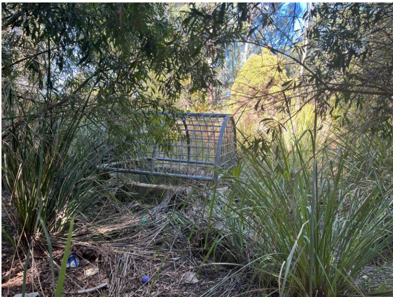
Figure 83. Overflow pit with raised dome grate. Photo credits: Jack Mullaly.
