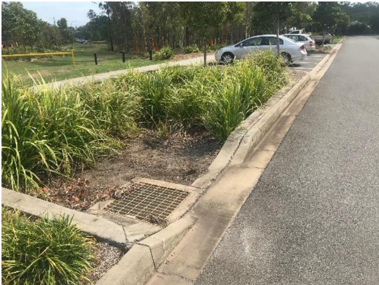
Figure 45. Poor example of an inlet and outlet located close to each other, where short-circuiting occurs. Photo credit: Brad Dalrymple.
