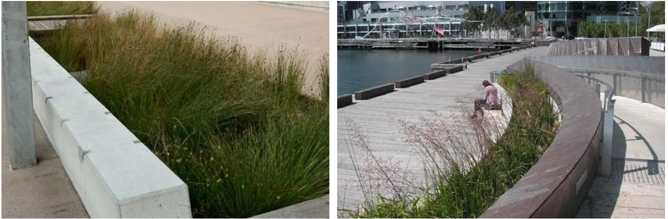
Figure 51. Well-designed bioretention system walls. Photo credits: left, Shaun Leinster; right, Robin Allison.
