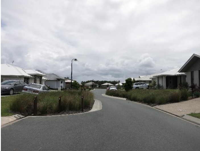
Figure 30. Collocation of bioretention with traffic calming. Photo credits: Paul Dubowski.
