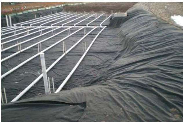
Figure 35. Bioretention system liner extended over embankments. Photo credit: Shaun Leinster.
