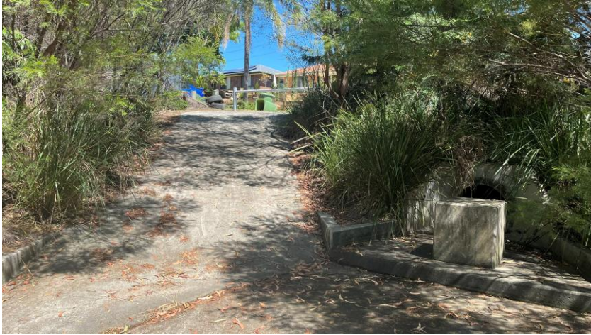
Figure 58. Well-designed and constructed maintenance access. Photo credits: Jack Mullaly.
