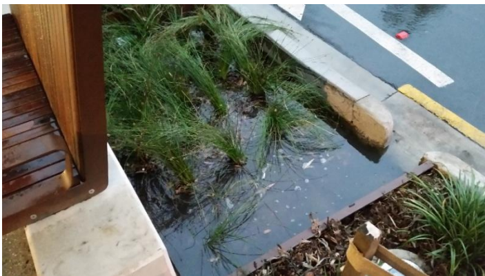
Figure 29. Streetscape bioretention systems receive inflows as surface flow. Photo credits: Jack Mullaly
