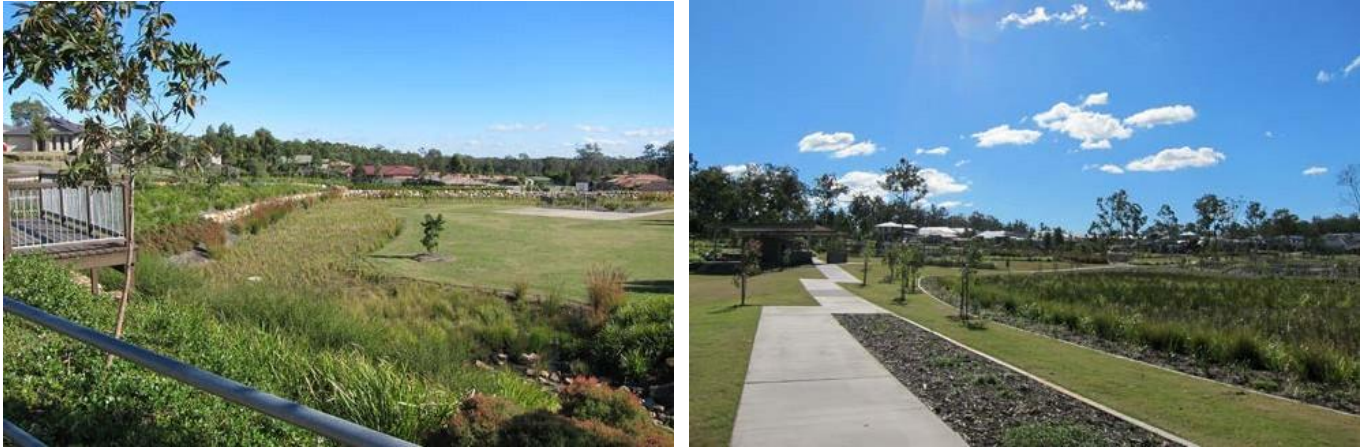
Figure 7. Examples of bioretention systems within and adjacent to parkland. Photo credits: top left, Shaun Leinster; top right, Jack Mullaly; bottom (left and right), Jack Mullaly.
