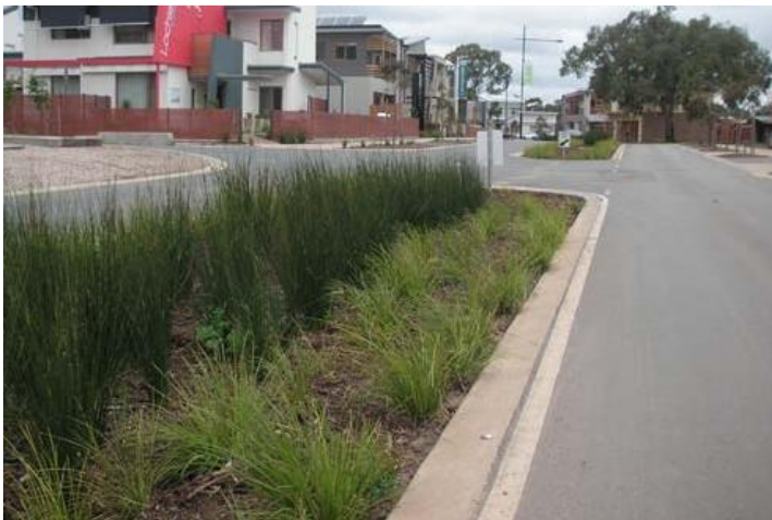
Figure 64. Flush kerb to promote distributed flow into the bioretention system. Photo credits: Robin Allison.
