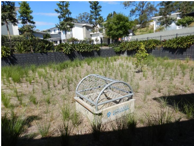
Figure 49. Unacceptable use of walls in bioretention systems. Photo credits: Paul Dubowski.
