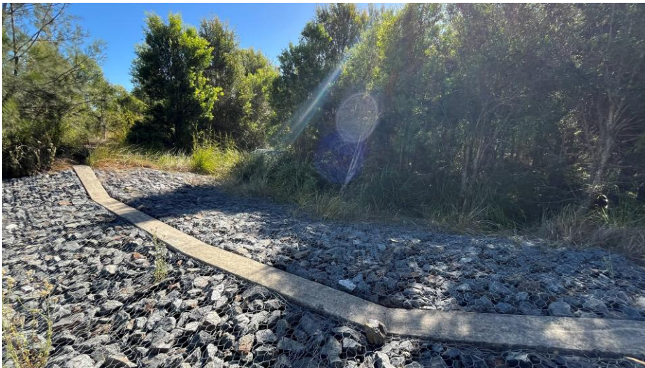
Figure 85. Example overflow weir. Photo credits: Jack Mullaly.
