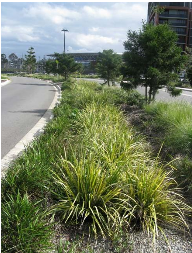
Figure 5. Examples of bioretention systems in the streetscape. Photo credits: top left and top right, Shaun Leinster; bottom left, Jack Mullaly.
