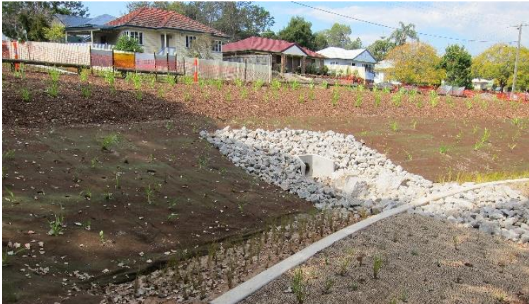
Figure 72. Level spreader. Photo credits: Jack Mullaly.
