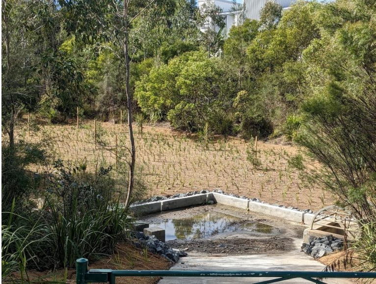
Figure 44. Good example of an inlet and an outlet located close to each other. Photo credit: Andrew Cook.
